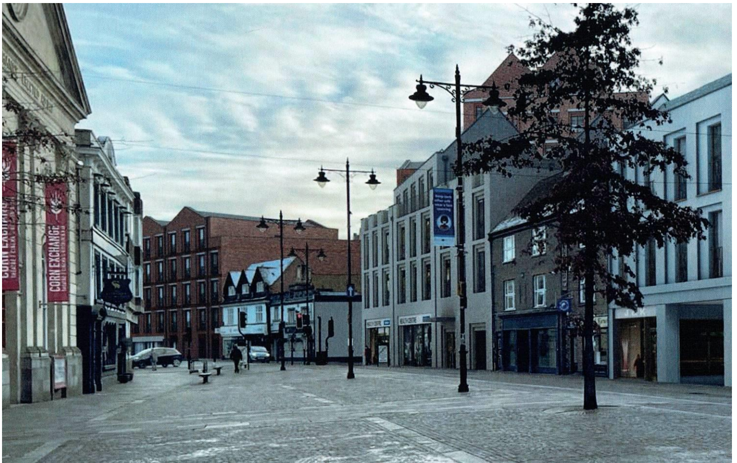
View towards Cheap Street from the Market Place showing Block C in the distance, next to “Save the Children”, part of Block G to the left of the tree, and part of Block A behind the tree.
