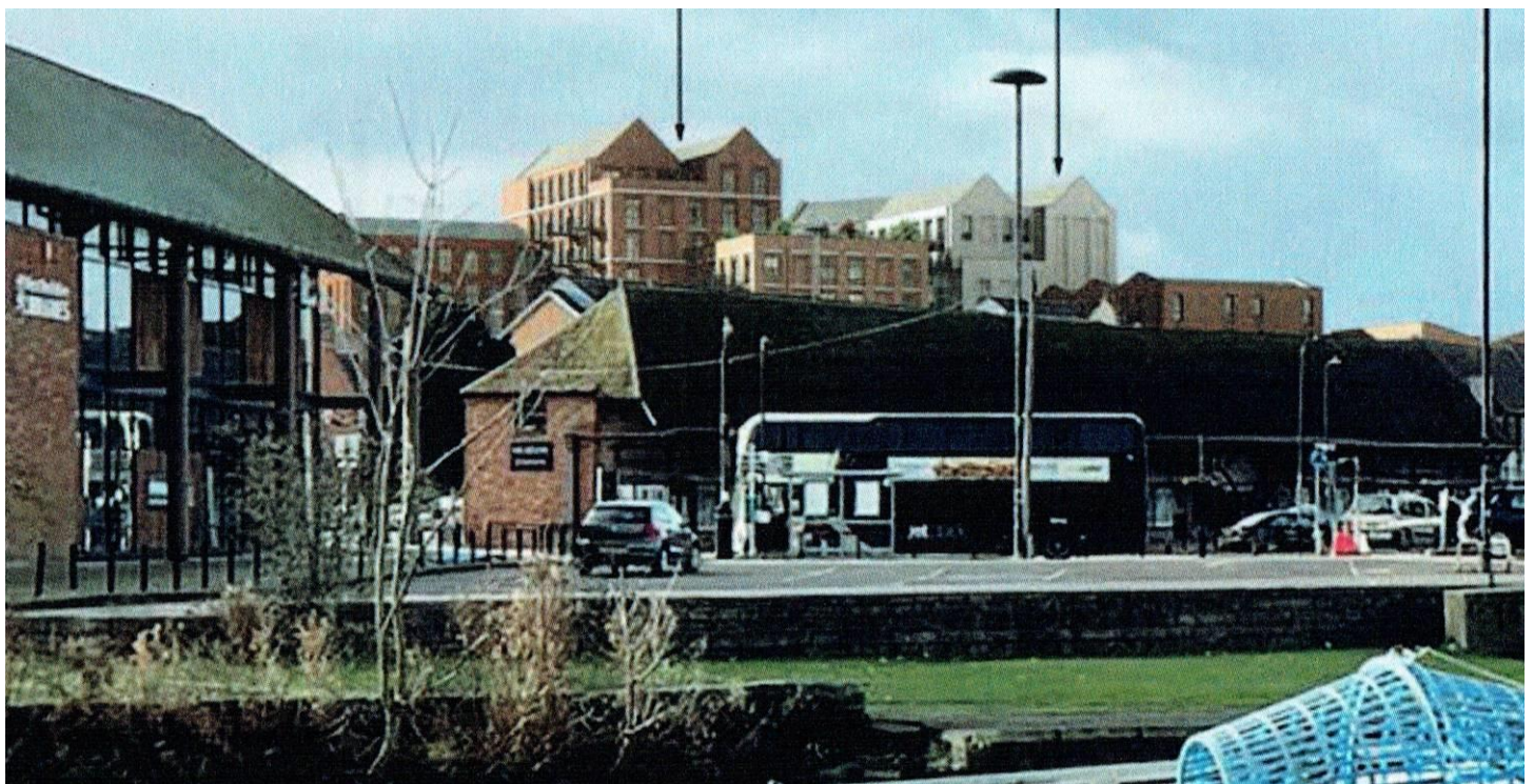
View South across Newbury Wharf , with Blocks A and B as the tallest visible behind West Berkshire Museum.
