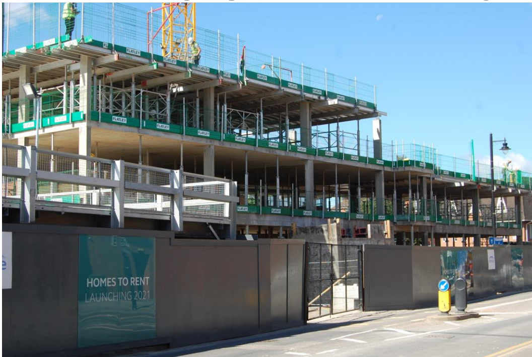
The current state of progress of the Market Street development
